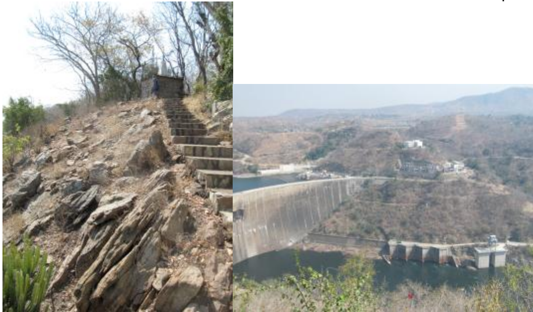
Figure 13 a and b: Banded Kariba Quartzite with weathered gneiss dipping downslope to the gorge, and view to the north-bank with new civil developments relating to the two new 180MW generators.
