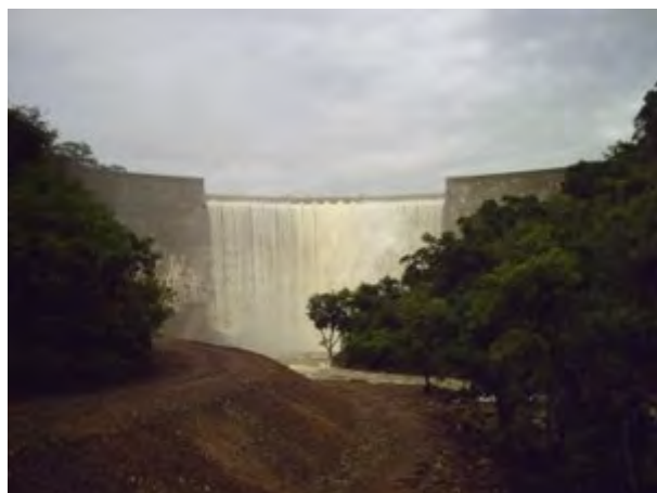
Lucilia Poort Dam, Shurugwi – Unki Mine Water Supply
