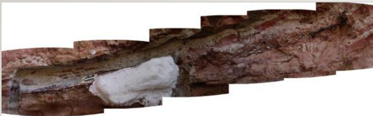
A slot prepared, blocks are jacketed and removed.
